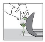
Clean the seam area, remove the release paper from the cover tape, press on and connect it to the membrane by rolling it on.
